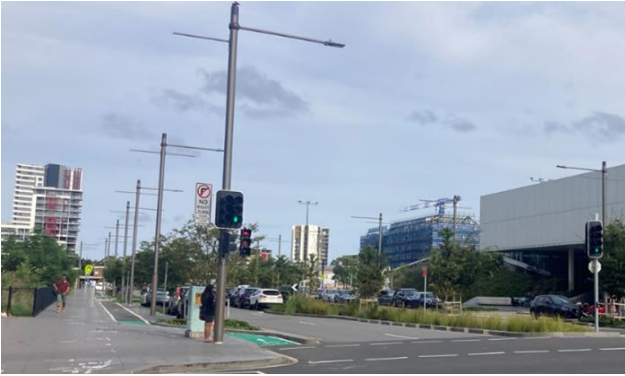
Picture 7 View looking along Zetland Ave with Gunyama Park Aquatic and Recreation Centre to south
