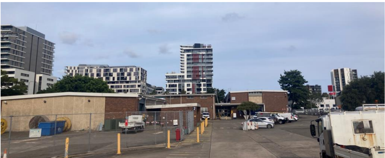
Picture 4 Two-storey building on western part of the site
